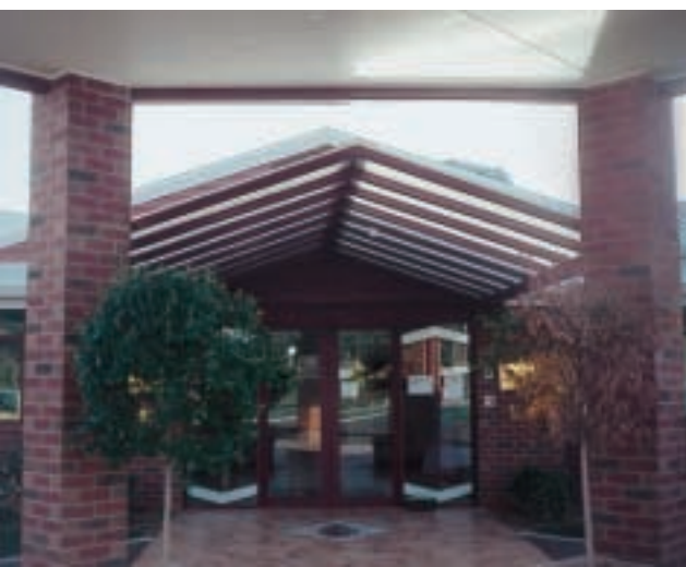
Underground cabling in walkway areas required only a single Category 5 cable to provide a C-Bus communications link.
